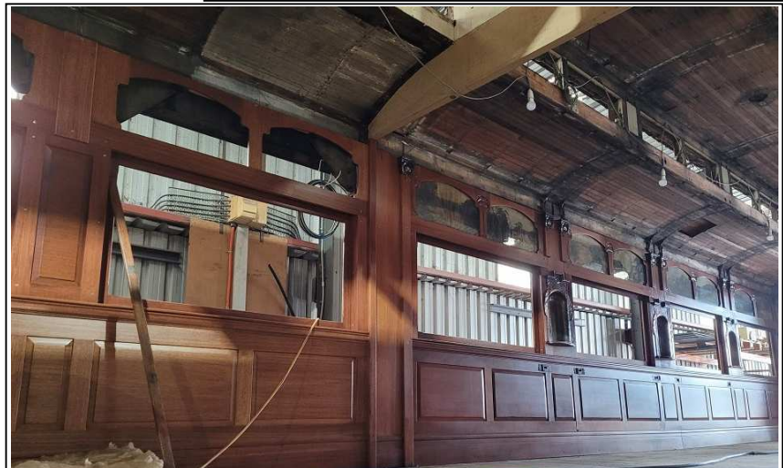
→ The Queensland Cedar panels have been sanded back and refinished.
